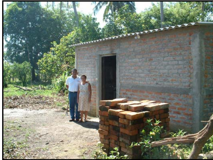
Alba Magda Miranda, an Integral client, near Zacatelocua, El Salvador, in front of her new 48m2 home. She built the house with a $1,740 loan from Integral, plus $750 of her savings. Note the horizontal cement reinforcement to protect against earthquakes.
